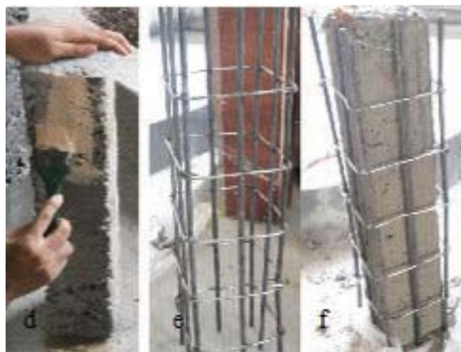
**Fig 1.** a. Reference Sample. b. Surface roughening c. Sand blasting. d. Application of epoxy bonding. e. Jacketed framework. f. Application of jacket before casting
