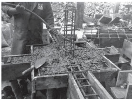
Fig 7. Concrete Casting of the Models
