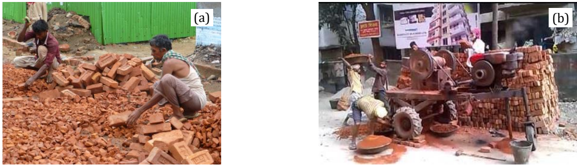
Figure 3: Brick crushing method: (a) manual process, (b) machine crushing
