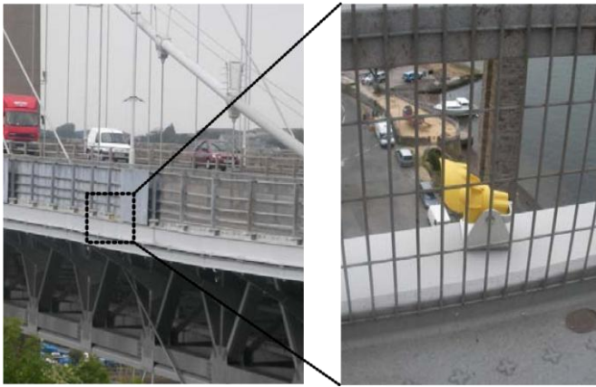
Figure 7: Reflector in bridge deck [25]
