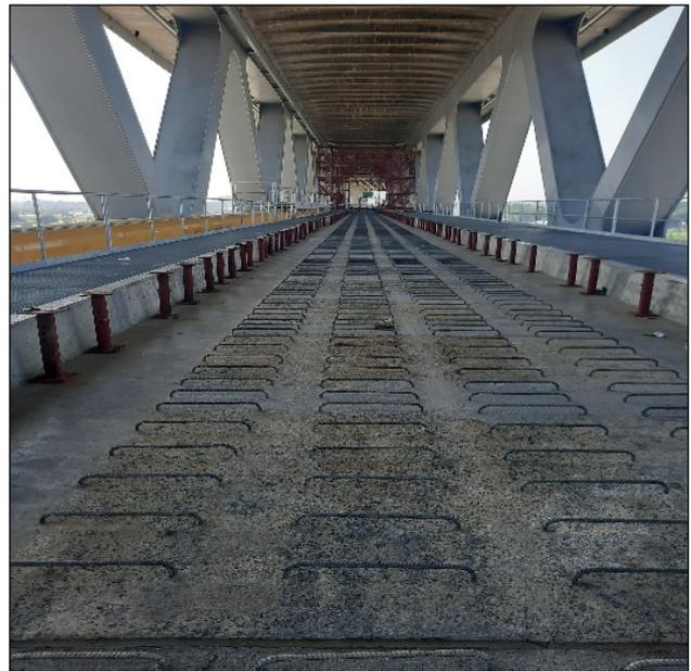
Figure 2: Shear Connectors provided at the lower deck of the Padma Bridge
