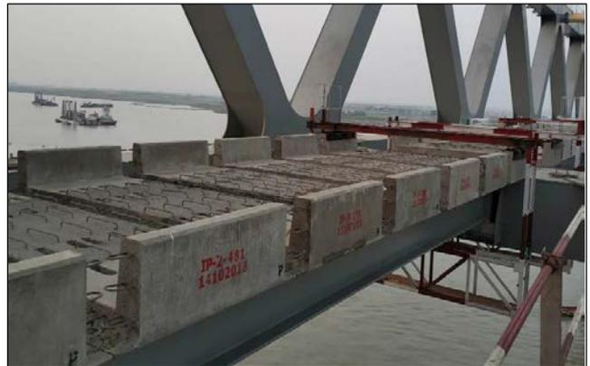
Figure 13: Long Sleeper Embedded BLT over Padma Bridge
