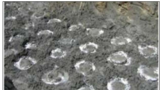
**Figure 9:** Cement Mixing Piles after construction
