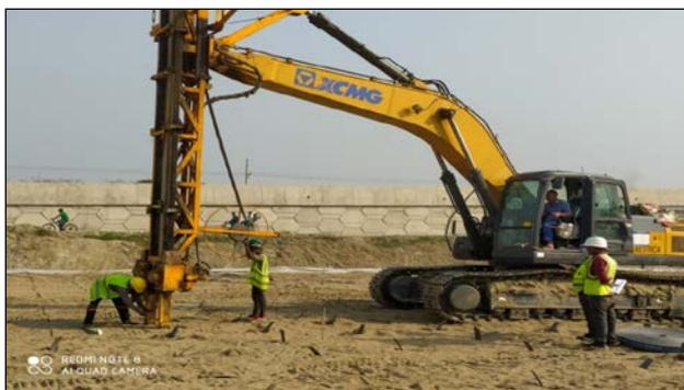
**Figure 7:** PVD being installed in the embankment
