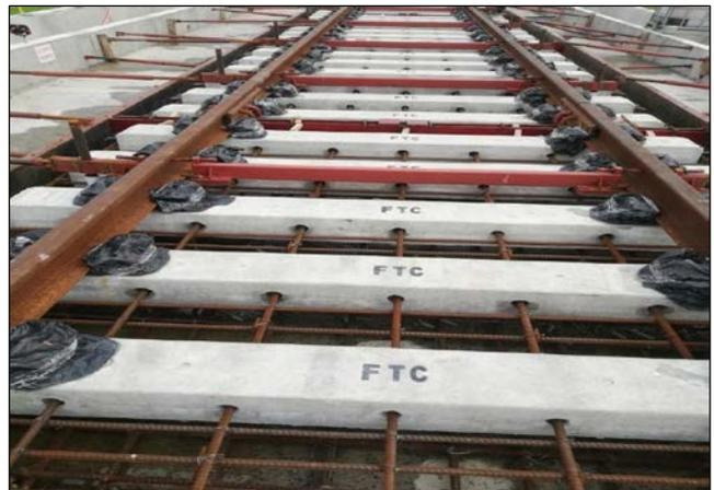
Figure 14: Semi precast cast in situ BLT
