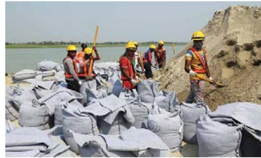
Figure 9: Dumping of Geobags on the lower slope
