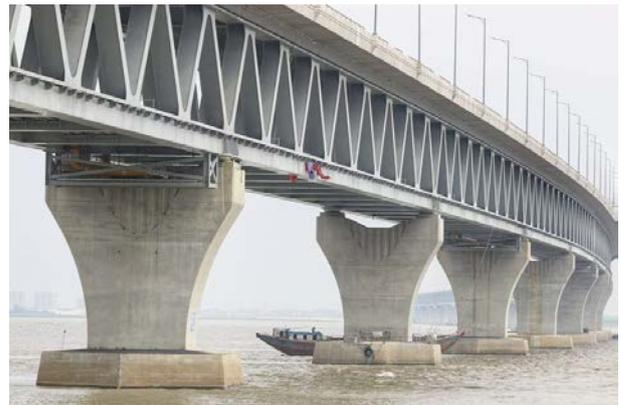
**Figure 7:** Provision for a dual gauge double-stack container freight rail line along the lower deck.
