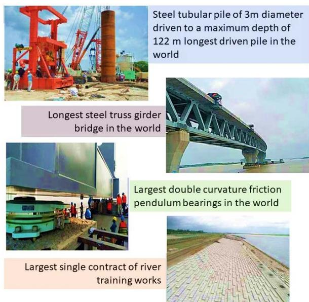
**Figure 3:** Record-breaking works of Padma Bridge Project (*Padma Multipurpose Bridge Project, 2022*)
