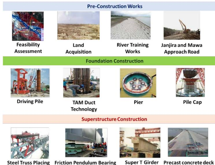
**Figure 8:** Padma Bridge Project Construction Processes
