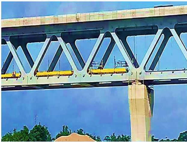
Figure 2: Gas pipeline and telecommunications cables in Padma Bridge (Padma multipurpose bridge project, 2022)
